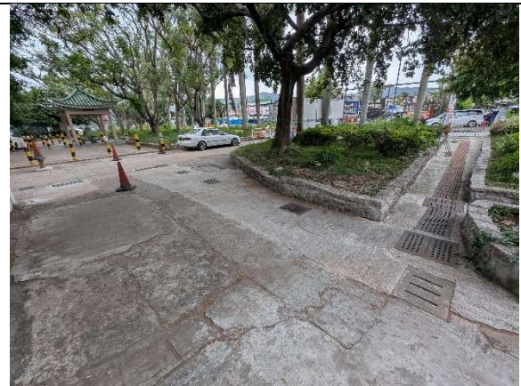
Plate 4 – Existing channels outside the southern boundary of the Application Site conveying surface runoff away.
